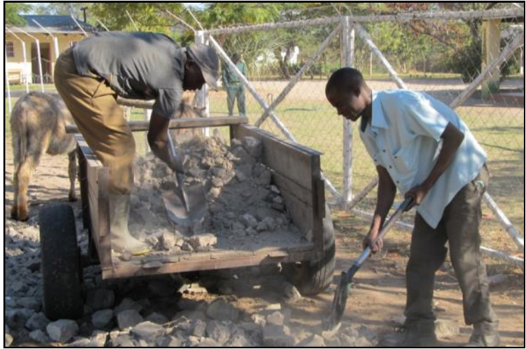
Starting the road repair work.
